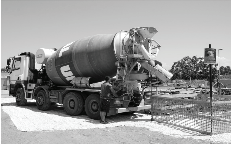
Fig. 2. The washout area
