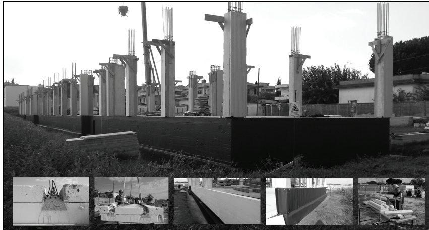
Fig. 1. Insulation of heat bridges
